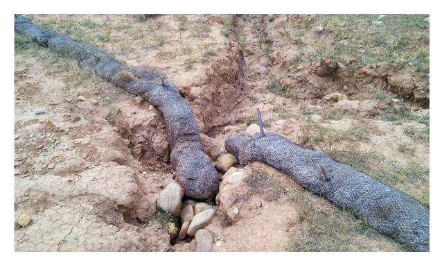
**Figure 5.** Failure of straw wattle, leading to rill and gully erosion. Proper installation is necessary to avoid failure. In this case, wattles may not be sufficient to prevent erosion and other measures are needed.
