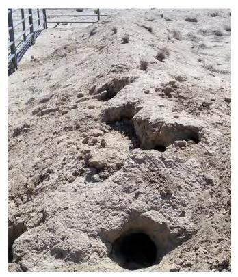
**Figure 11**. Earthwork berms are easily damaged by wildlife or other activities at a well site, and greatly increase the risk of berm failure in case of a spill, which can contaminate interim reclamation.
