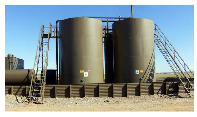
Figure 12. Metal berms are easier to maintain and more cost effective in the long term.
